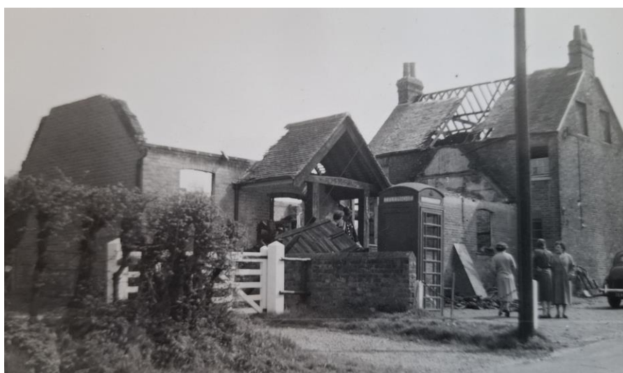
Sunday, 12 th April 1959 – the morning after the fire
